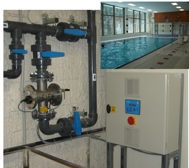
AlfaLine UV medium-pressure 'in-one-line'-UV system in therapy pool. Courtesy: bestUV
